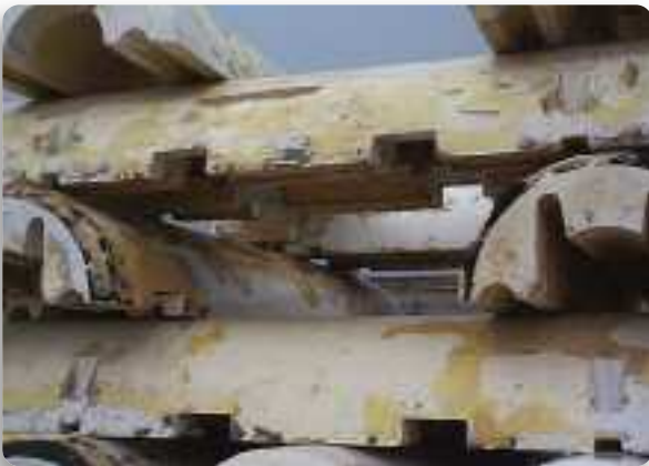
Drilling riser buoyancy modules before and after repair
